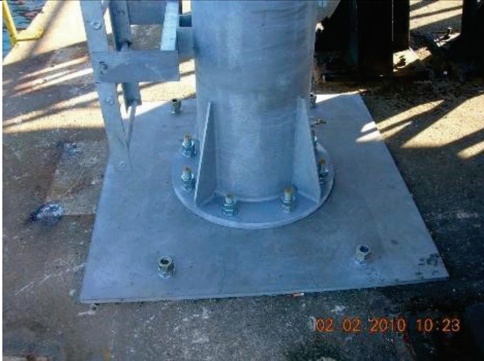
GAETA (LT) – PARTICOLARE STRUTTURA SPECIALE DI ANCORAGGIO IN ACCIAIO (ESTRADOSSO BANCHINA)
